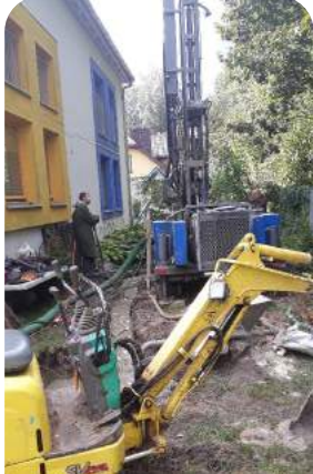
▲ Drilling boreholes for the ground heat exchanger.
