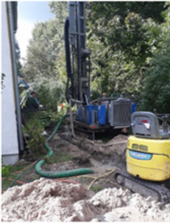
Ground heat exchangers
