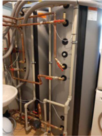
Buffers in boiler room
